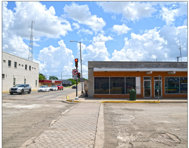
UNDERUTILIZED COMMERCIAL BUILDING, PINE STREET AND 10TH STREET
